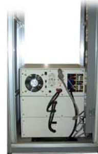
View of SU Plus installation PG2604, battery pack shall be connected easily to rear side of the UPS. The height of UPS's electronic module is 4U, and PG2604 is 3U.
